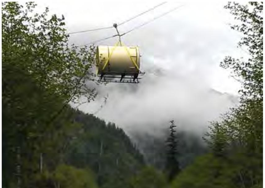
FIGURE 3: Transporting the Shaft Liner to the Top of the Surge Shaft
