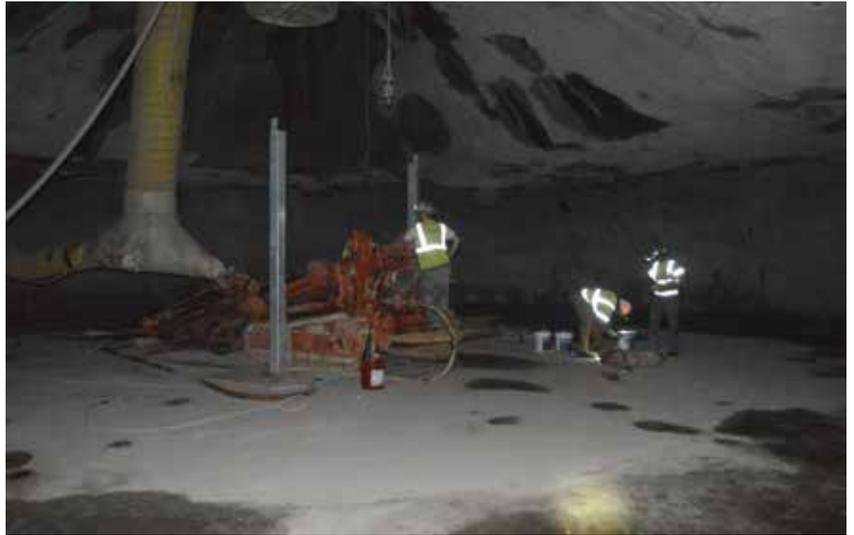
DRILLING GALLERY: Matt Bauer prepares the airtrack for installation of the ground support.
