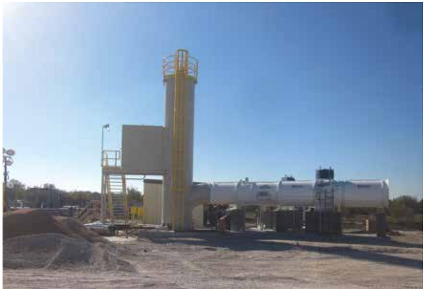
**ESCAPE HOIST:** Emergency Escape Shaft with Hoisting System and Dual Fan with air lock.
