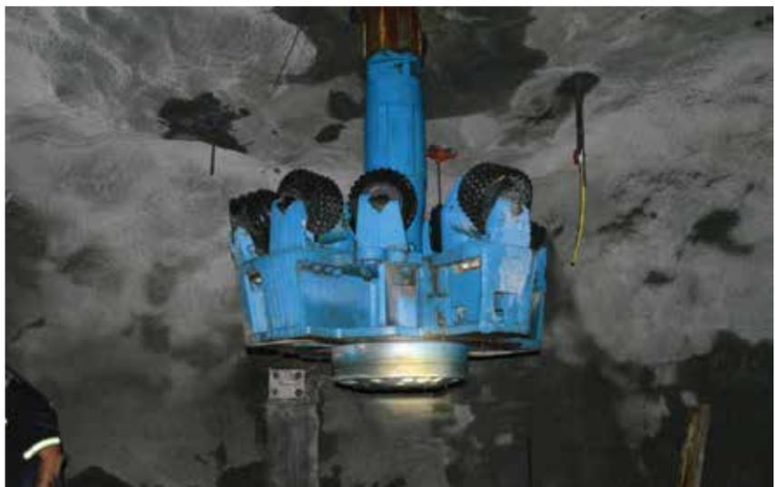
EMERGENCY ESCAPE/VENT SHAFT: Reamer head is attached and raised to start reaming the Emergency Escape Shaft.
