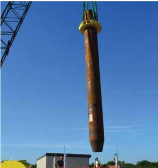
**EMERGENCY ESCAPE SHAFT:** First piece of casing is lowered into the Emergency Escape Shaft.
