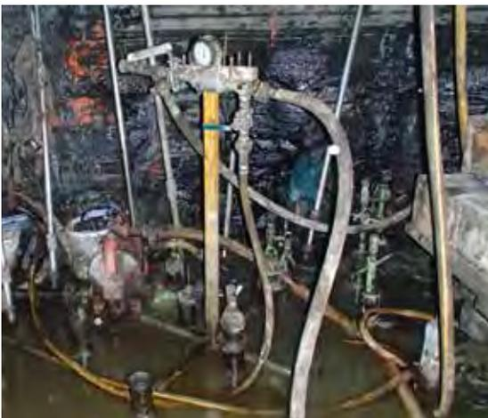
MAIN ACCESS SHAFT: Typical pre-grouting manifold set up on Shaft floor.
